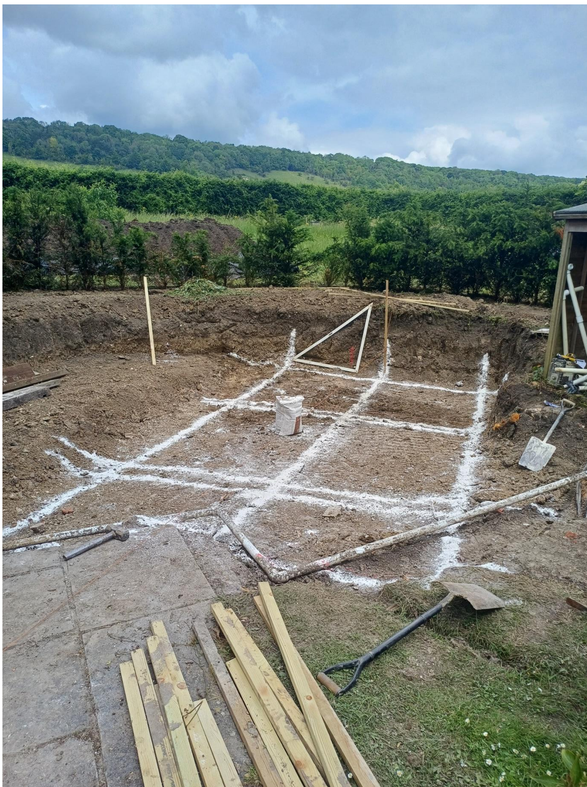
Plate 2. Setting out (looking North)
